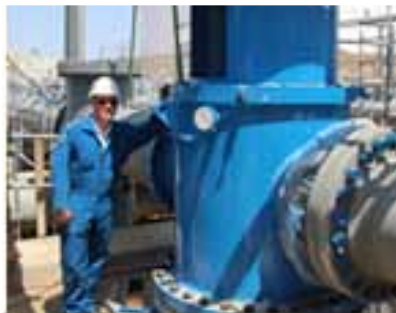
Vertical pump being serviced.
