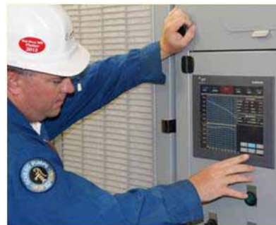
Provides operations with a "window" into real time pump performance and operation. Dynamic pump flow/head/power curve changes with speed.
