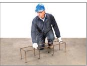
Install new rebar cage (new installation) or expose existing rebar (existing installation).
