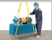
Install Polyshield® Foundation complete with pump and motor over rebar.
