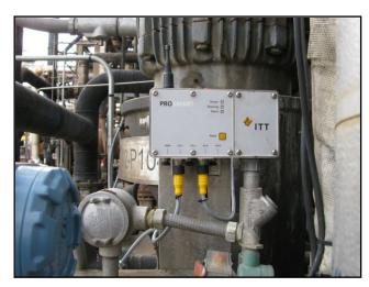
By adding an ITT ProSmart condition monitoring system, United Refining can use real-time data to prevent pump failures.
