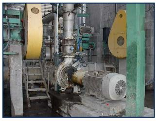
By adding an ITT PumpSmart controller to a third-party pump, the Plant Performance Services team helped achieve dramatic cost savings in the mill's towerpumping operation.
