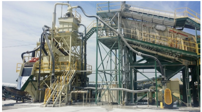
Crushed Stone Plant
