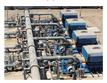
Twenty Goulds 3600 API pumps propel seawater 90 miles from the Pacific to the Esperanza copper mine, while 14 ITT employees are on site for daily pump inspection, ProSmart data monitoring, and implementation of other Plant Performance Services (PPS) assessment recommendations.
