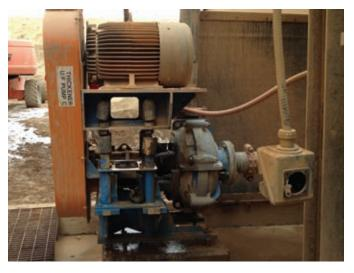
The half-straddle motor mounts allow easy access to packing box area without dismantling the motor.
