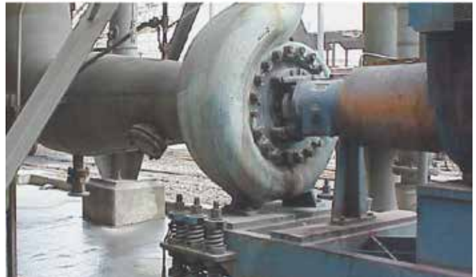
Model 3180XL on difficult high temperature service. Spring-mounted baseplate provided to compensate for thermal expansion.
