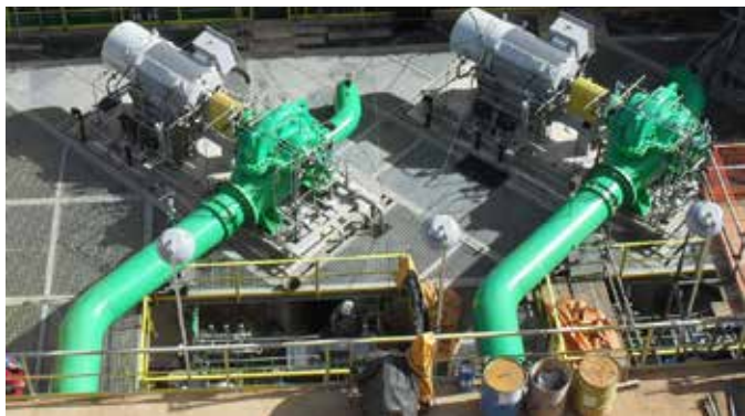
Refinery Cooling Tower Service (Brazil)
