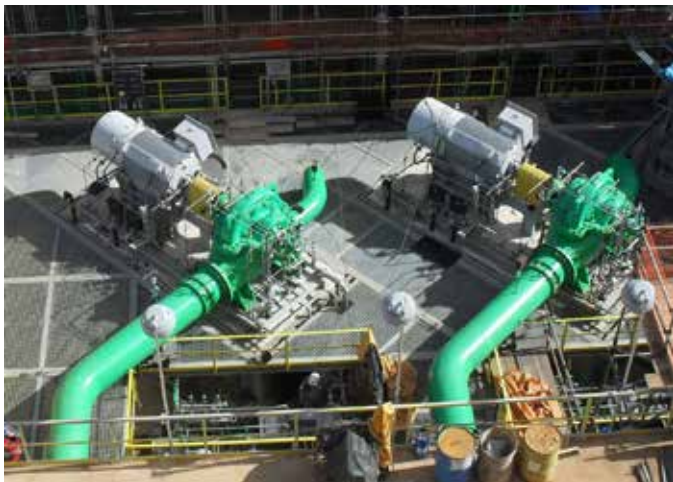
Refinery Cooling Tower Service (Brazil)
