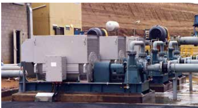
Gold Tailings Pumps in Australia - 3700 4x6-19
