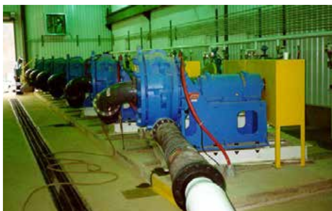
High Pressure Design available for series pumping needs in coal processing plants.
