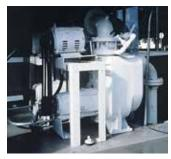
Trash Hogs are utilized in remote sewage lift stations to pump municipal waste from outlying residential areas to the local treatment plant. Here, Trash Hogs are being driven by overhead belt drives to conserve lift station space. Service will be performed by removing the rotating element to the rear as typical suction piping restricts access to the front of the pumps.
