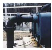
In this installation, two 3" Trash Hogs are being used to control the level of the liquid in these settling ponds. Liquid level controls in the sump determine whether either or both pumps are needed to maintain proper pond level. Trash Hogs were chosen due to their reliable priming capabilities.
