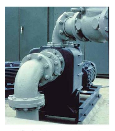
Here, one of several 6" self-priming Trash Hogs is being used to pump process waste at an industrial treatment plant. Trash Hog was specified and installed due to its ability to pass a 3" diameter solid and prime and reprime a 15 feet static suction lift.
