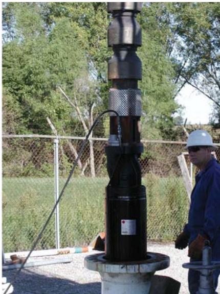
125HP proves to be a tight fit into the pump caisson.
