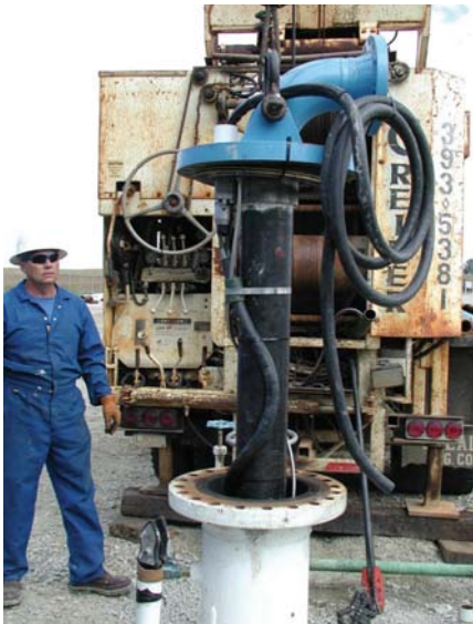
Head/Discharge elbow lowered onto caisson.
