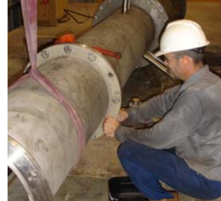
Harry Mathers bolts columns together.
