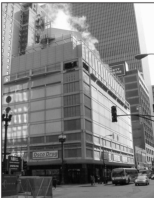
Exelon plant #1 in downtown Chicago can produce and store over 5 million pounds of ice daily.
