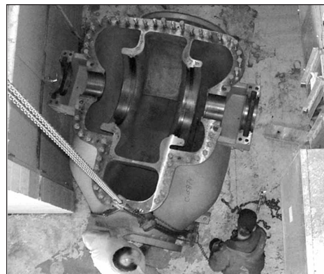
The casing is lifted to the second floor of plant #1.
