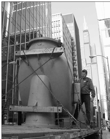
ITT PRO Services personnel prepare to unload the lower casing half.
