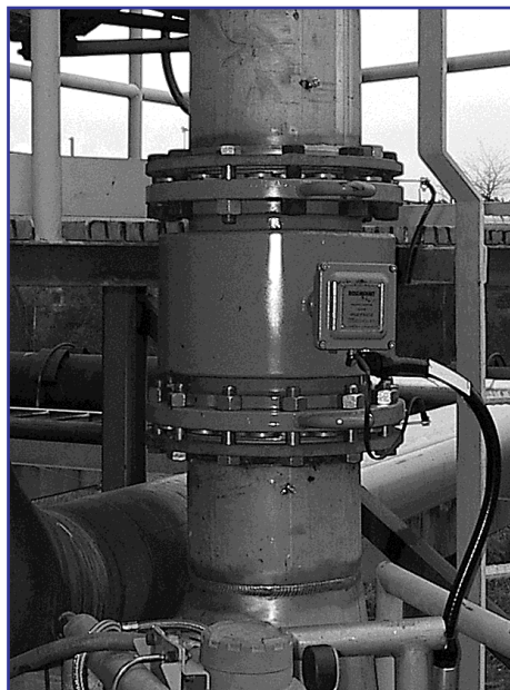
Figure 2. Flow tube replaces inefficient control valve.
