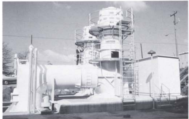
Vertical Wet Pit Column Pumps offer valuable floor savings since the driver is mounted directly above the pump.
